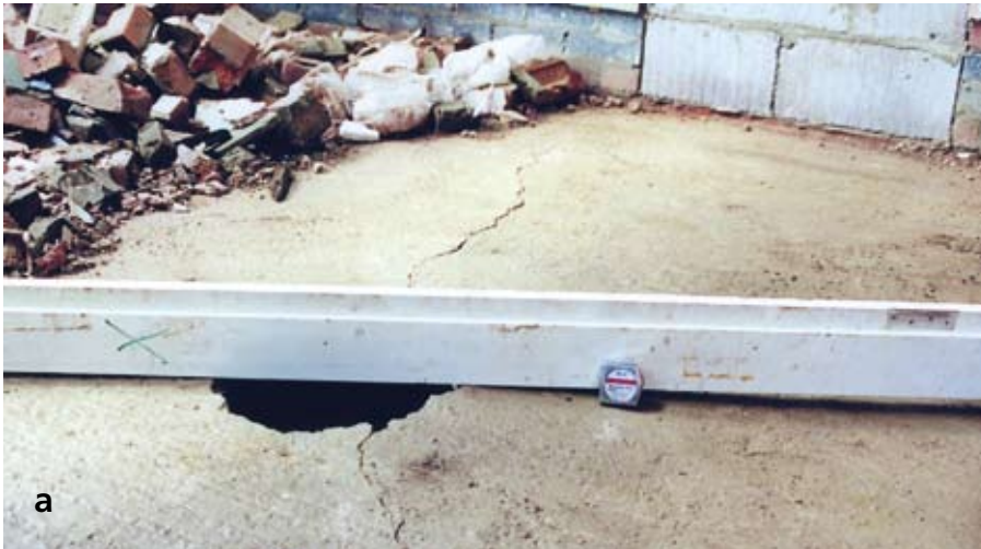
Figures 7(a, b & c): Sulfate-attacked oversite concrete that was laid over plaster contaminated brick rubble beneath a suspended wooden floor (here removed together with the sleeper walls). (a) An improvised straight edge shows some 50 mm doming of the oversite concrete that lifted brick sleeper walls and wooden floors.
