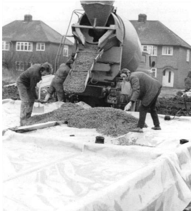
Figure 4: Laying of concrete in the mid 1970s on a 300 micron damp-proof membrane that has been placed over hardcore in the foundations of a house.
