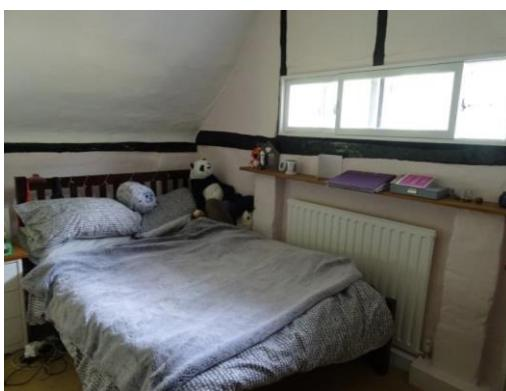
The walls and ceilings are plastered, finished with a mixture of lining paper and emulsion with no structural cracking noted. General distortions were noted to the ceiling where the plaster finishes have begun to de-bond, however not considered unusual for the age of the property.
