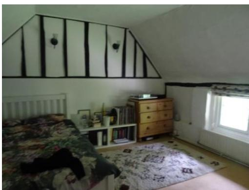
The walls and ceilings are plastered, finished with a mixture of lining paper and emulsion with no structural cracking noted. General distortions were noted to the ceiling where the plaster finishes have begun to de-bond which is not considered unusual for the age of the property.
