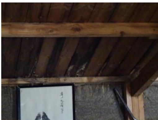
The roof has been supported on timber trusses which were noted to be structurally sound with no deflection noted.
