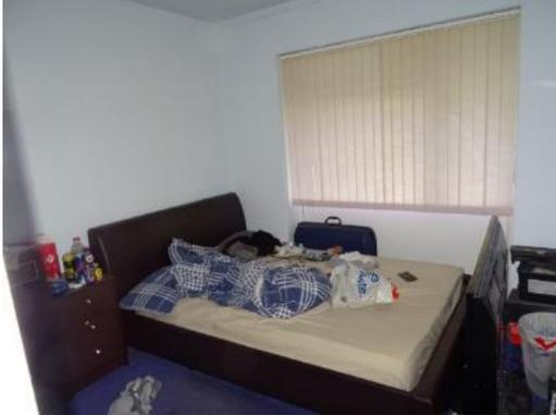
The walls and ceilings are plastered finished with emulsion. Slight board cracking was noted to the ceiling however of no significant concern.
