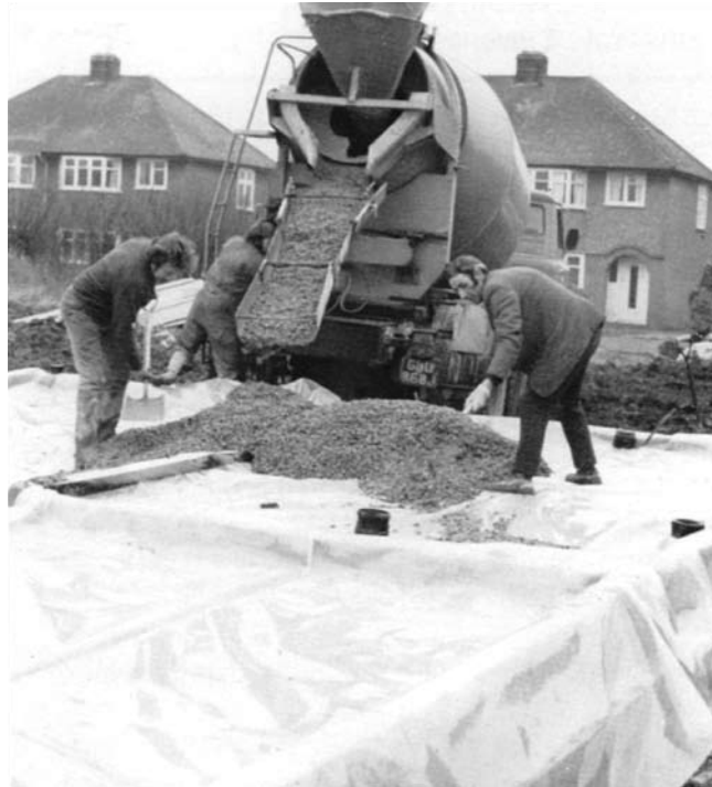
Figure 4: Laying of concrete in the mid 1970s on a 300 micron damp-proof membrane that has been placed over hardcore in the foundations of a house.
